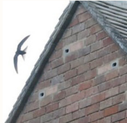
'Universal bricks' integrated within the building's fabric.
