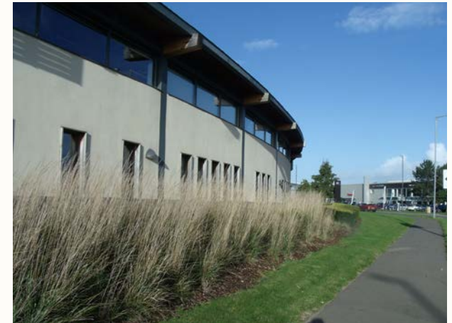
Hitachi Novuna Vehicle Solutions building in Trowbridge
