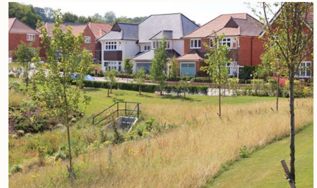
Generously planted Sustainable Drainage Systems within Marleberg Grange, Marlborough
