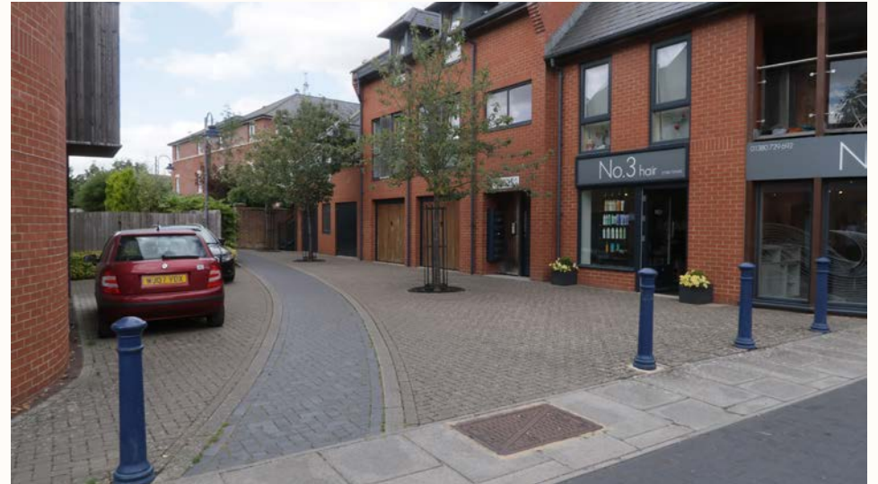
Attached built form and mews, Snuff Street, Devizes
